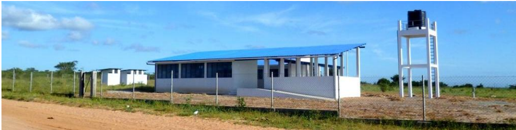
Figure 4. Newly constructed health centre outside Mtiticoma
