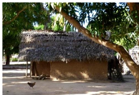
Figure 3. Typical rural house in Moma District
